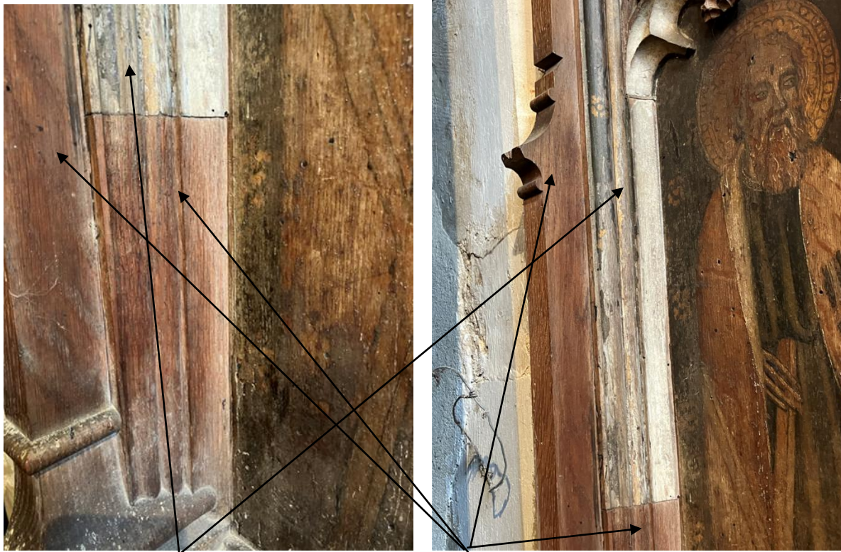
Combination of original framework and Victorian reconstruction.
