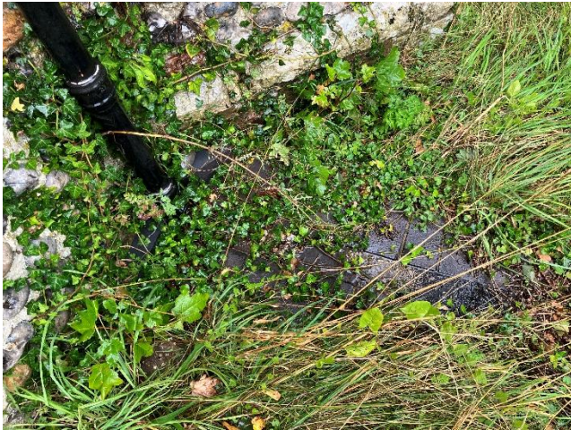
Debris and vegetation should be removed from the blue brick channels and grates and surface water drains.
