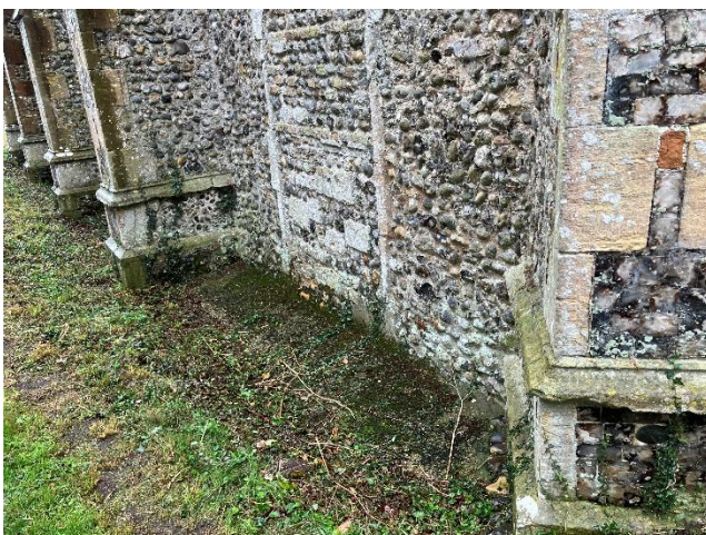
Foliage should be removed from the soakaway.
