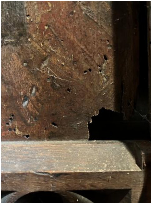
Damage and loss to the bottom right corner of panel number eight and the surrounding timber immediately below.
