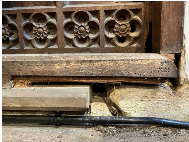
Damage and loss to the bottom right corner of panel number eight and the surrounding timber immediately below.
