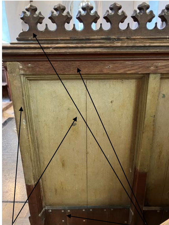
Combination of original framework and Victorian reconstruction.
