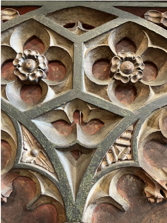
Original carved arches canopy.
