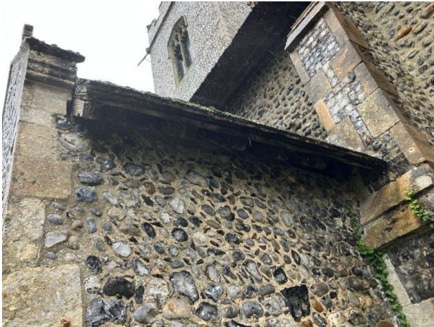
Sufficient overhang of eaves on the tiled roof, south porch.
