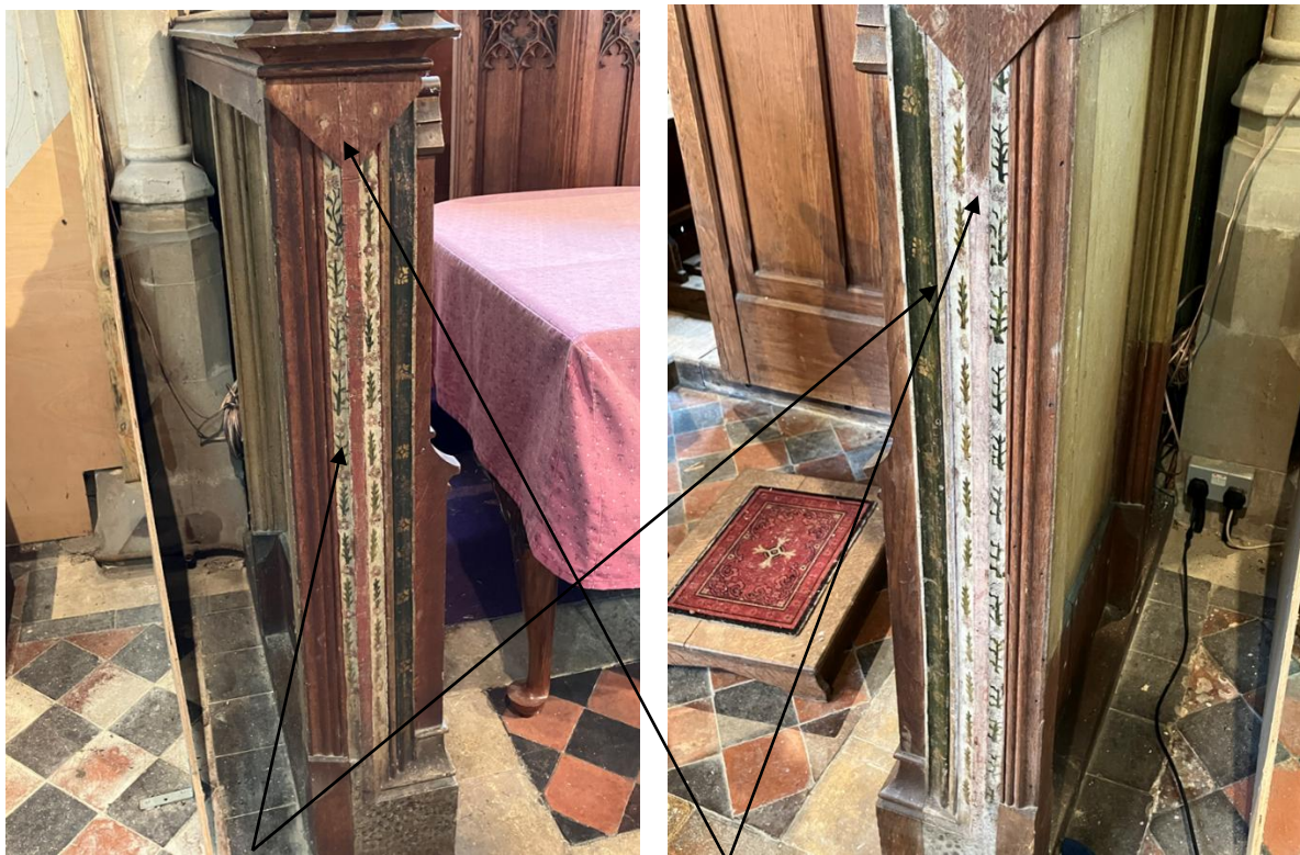
Combination of original framework and Victorian reconstruction.
