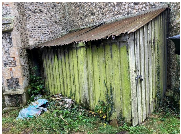
If no longer required it would be recommended to remove this shed.
