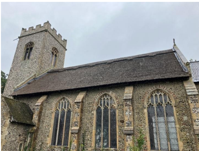
The new thatch on the nave roof is in good condition.
